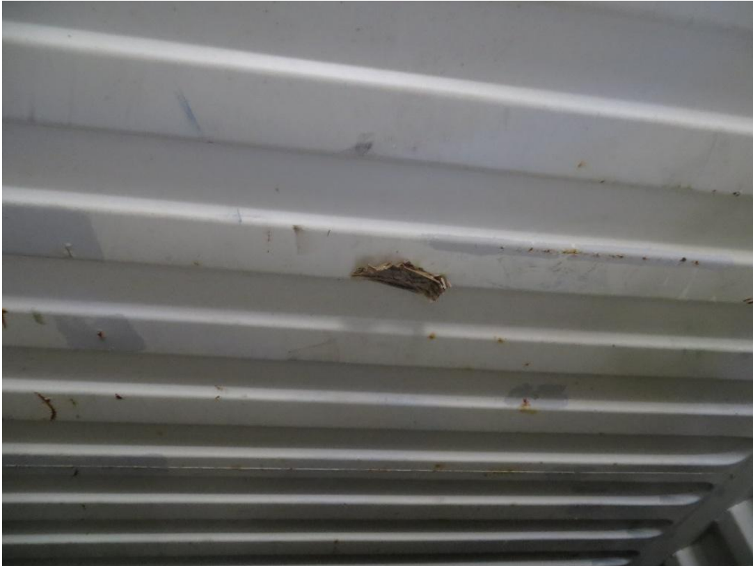
Tape over Hole in Container Roof(Excess International Tape) as found
