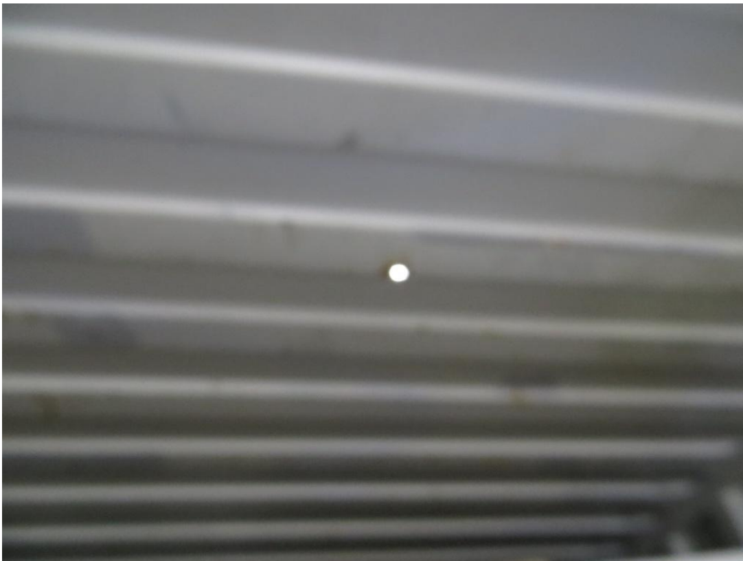
Hole in Container Roof
